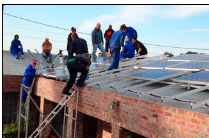
Installateurtraining 2012 in Kapstadt
